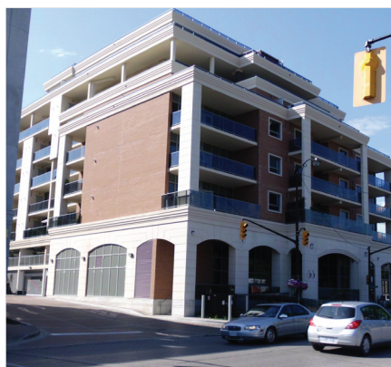
The river valley location called for a permanent waterproofing solution that would work with the tight schedule.
