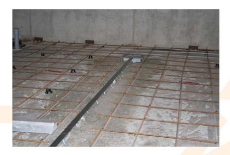
6. Once the concrete slab is firm, break out all metal tabs with a steel bar to ensure a continuous open slot. Remove the tape from the slot and, using the Paddle, clean out the U-drain and sump pit.
