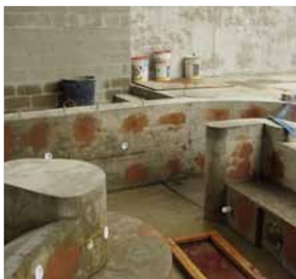
Construction of the 'lazy river' with Kryton pails in the background.
