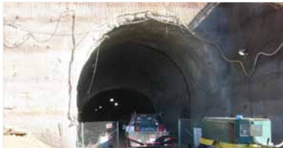
Shotcrete construction of the wine caves.
