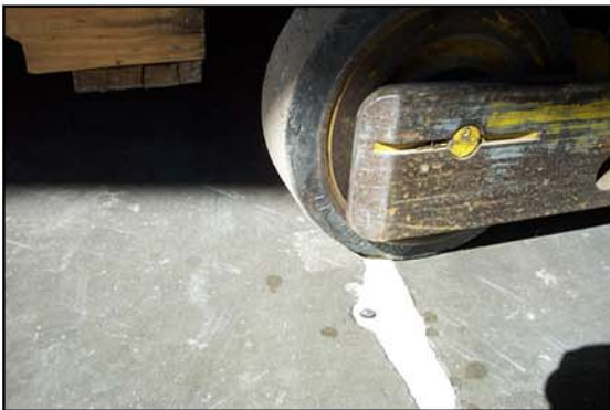
After 10 minutes, Floor Fix 10 is ready for heavy traffic
