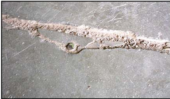
Before Repair with Floor Fix 10
