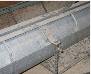
7. Once the U-drain is secured to the E-Z Mount Brackets and the appropriate floor height is found, tie rebar from the floor grid into the rebar on the U-drain assembly, for structural support. Cover the slot opening with duct tape.
