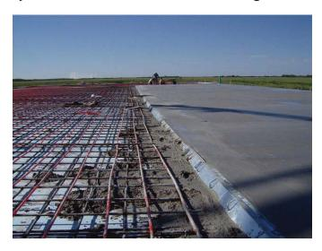
Once the concrete slab is firm, break out all metal tabs with a steel bar to ensure a continuous open slot. Remove the tapefrom the slot and, using the Paddle, clean out the U-drain and sump pit.
